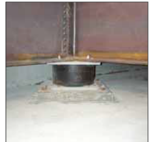
Seismic base isolator
